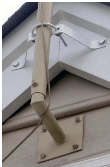
This is an image of the anemometer mounted to the north gable of the house.
